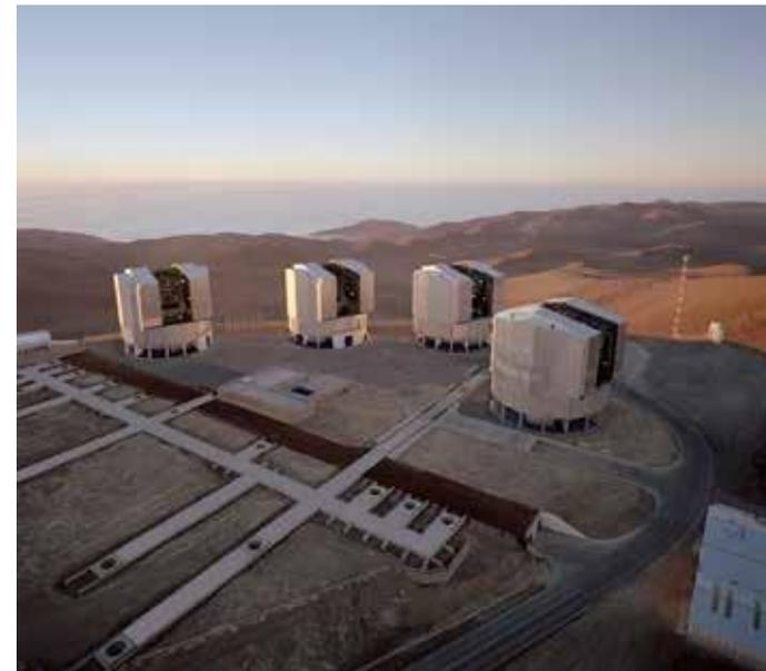
*8.2 m four telescopes of the Very Large Telescope of ESO (European Southern Observatory), usable as an interferometer (VLTI). Cerro Paranal (Chile)*
